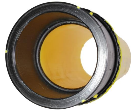
A joint welded according to the conventional technology
